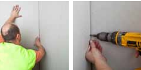
Secure Gyproc plasterboard in accordance with current Gyproc guidelines
