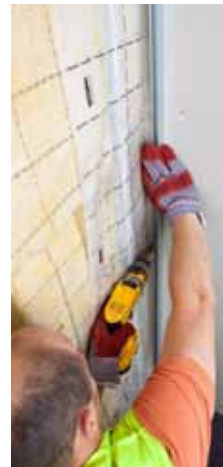
Fix U-channel to Gyproc plasterboard
