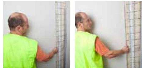
Secure Gyproc plasterboard to vertical U-channel
