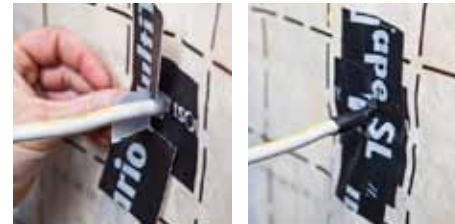
Attach Vario Multitape strips around the penetration as shown
