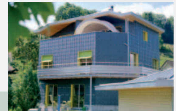
Office and residential building in Mosnang. Insulated with Flora natural hemp by ISOVER. Architect: Monika Mutti-Schaltegger.
