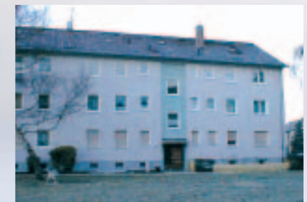
Multi-family house after energetic refurbishment
