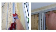
Extend extension piece until firmly into ceiling U-channel
