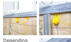
on window width, vertical supports may need to be inserted using Optima connector piece (fix base of vertical C-channel into floor U-channel)
