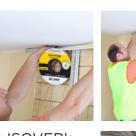
Fix ISOVER's doauble sided tape to the face of floor and ceiling **U-channel** (the use of Vario<sup>®</sup> DS Mastic is also recommended to seal any unwanted gaps)
