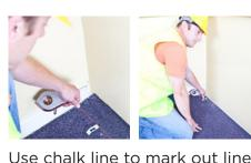
for floor U-channel - line marked is to front of U-channel
