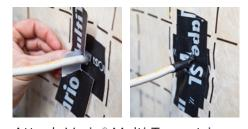
Attach Vario® Multi Tape strips around the penetration as shown
